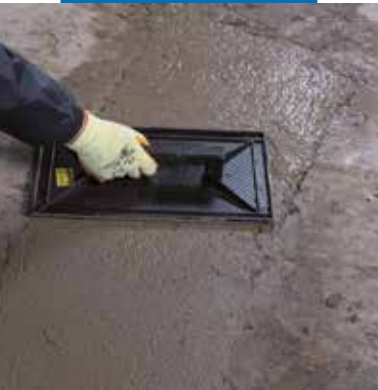
Talochage de Mapegrout SV Fiber
